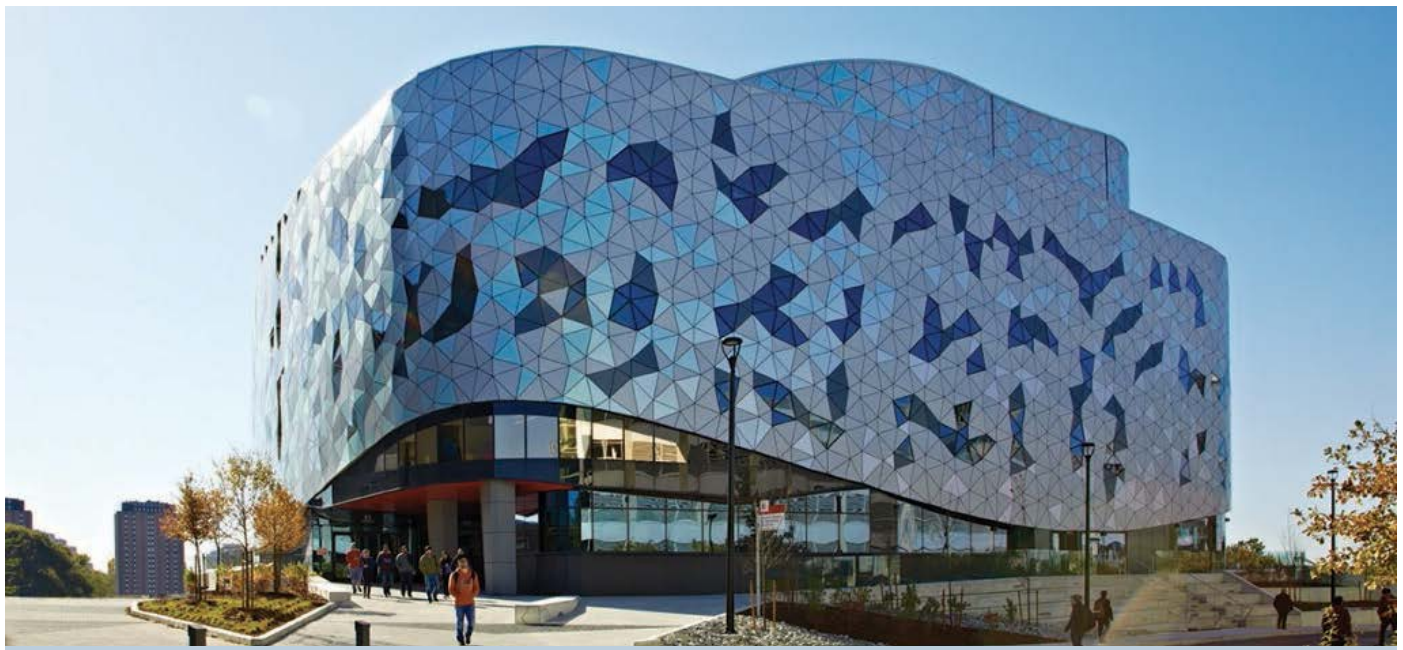
Bergeron Centre for Engineering Excellence, York University, ON
