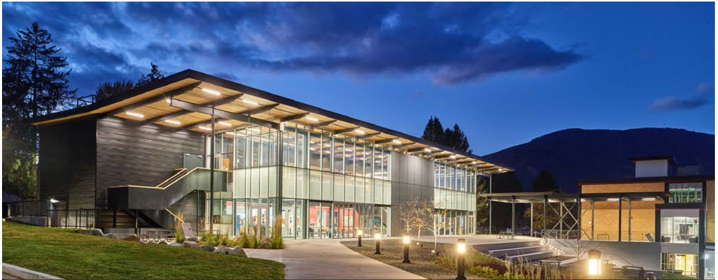
Student Commons Building Exterior, Selkirk College, BC
