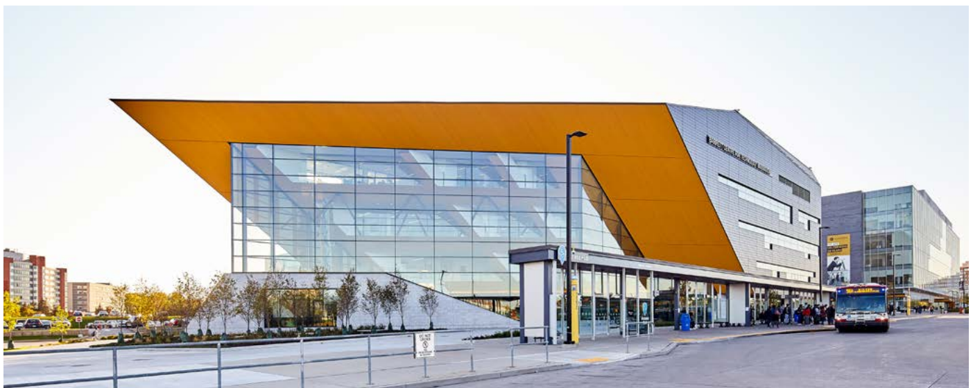
Below: Humber College, Barrett Centre for Technology Innovation
