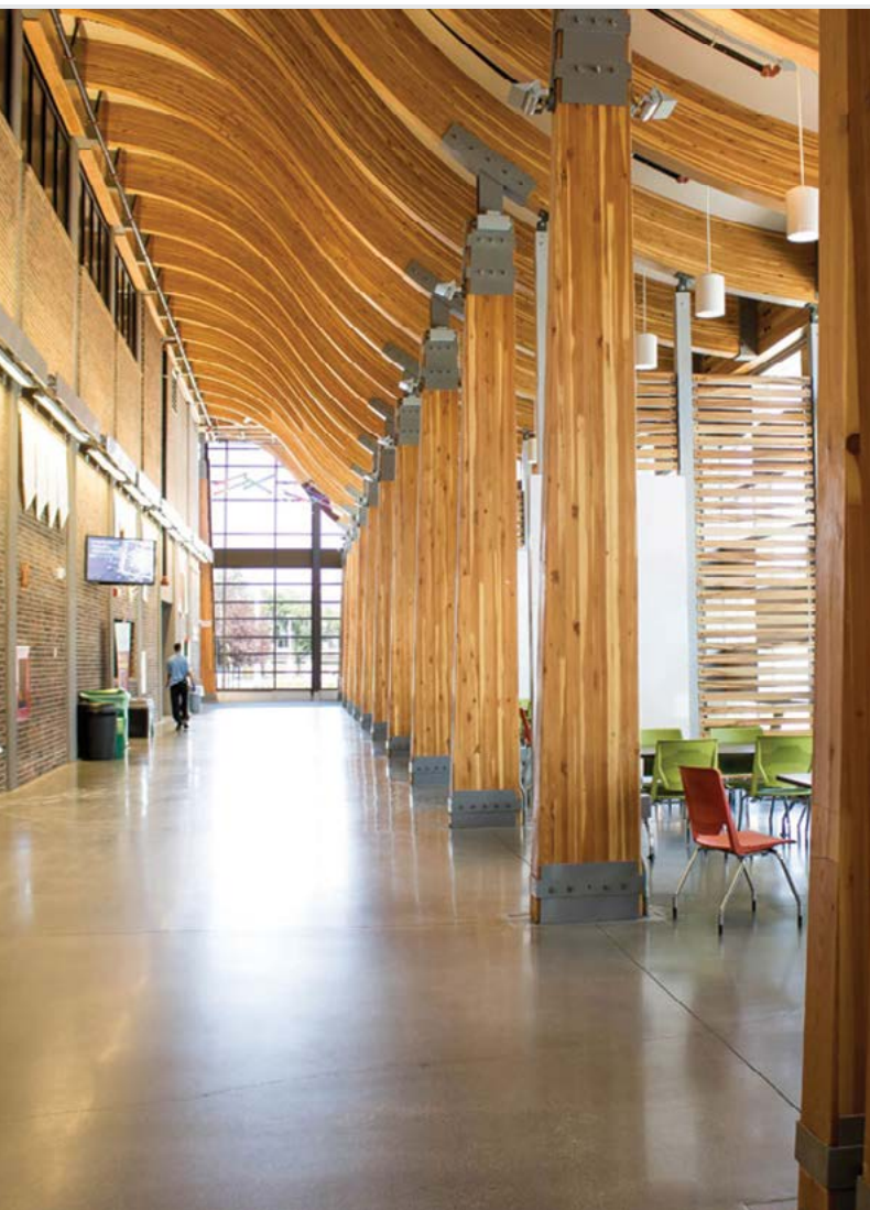
Thomas Riley Building, Southern Alberta Institute of Technology (SAIT), Calgary, AB. Photo: Woodpecker European Timber Framing.
