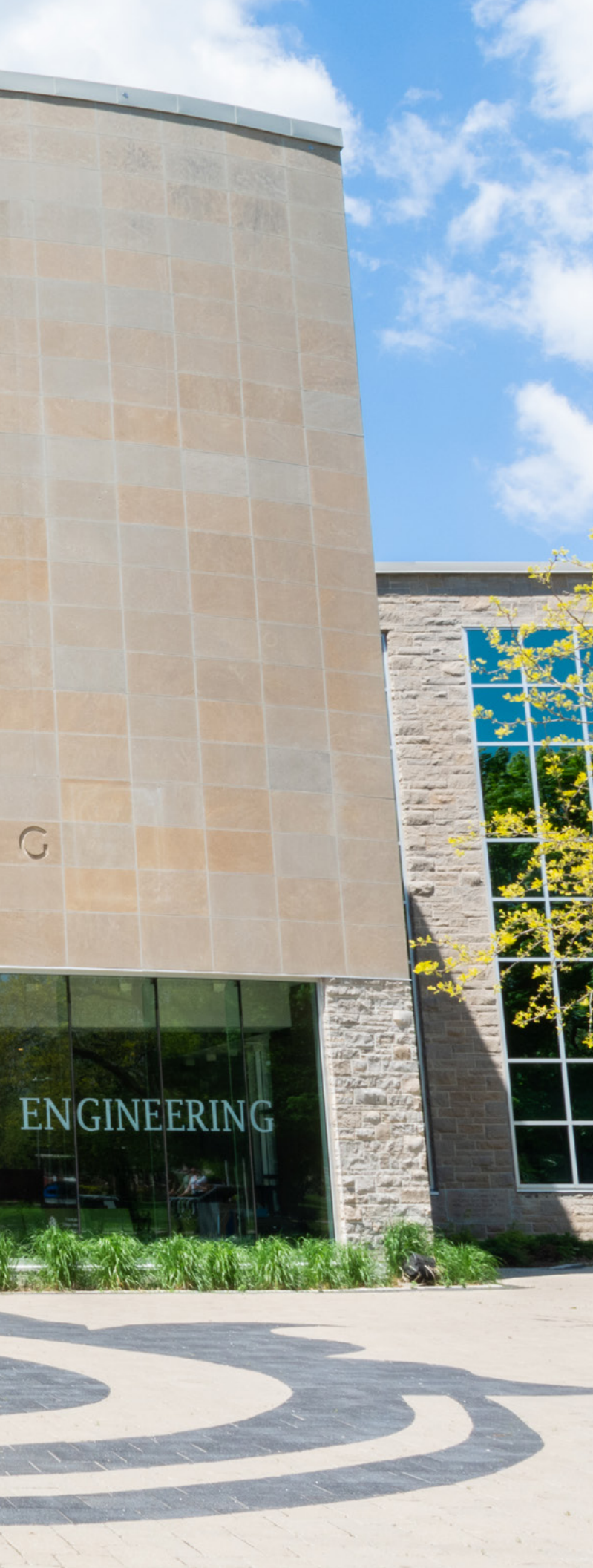
John Hodgins Engineering Building, McMaster University in Hamilton, Ontario
